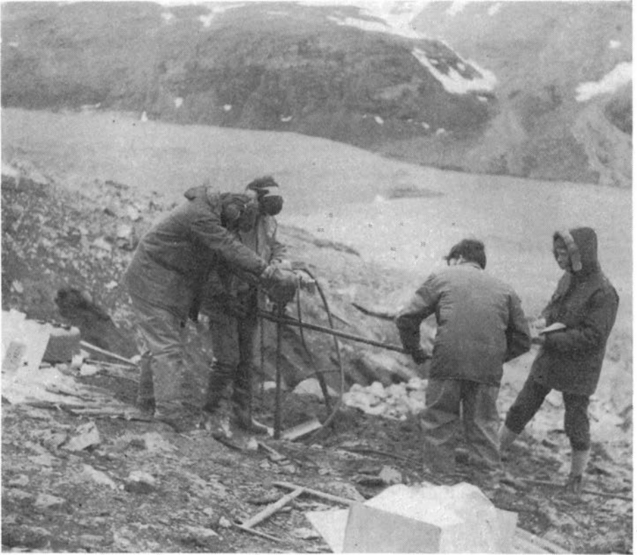
Fig. 1. Drilling on the north side of Ebbadalen. The man on the left is operating the drill, while the person in the foreground is holding the «jo-bar». The hole has been put down into loose cover, so a wooden board is being used as a stable platform and to provide an anchorage for the jo-bar chain. The water supply unit is not visible, but the connecting hose pipe can be seen, attached to the drill unit. A piece of guttering is being used to lead the returning water away from the platform.
