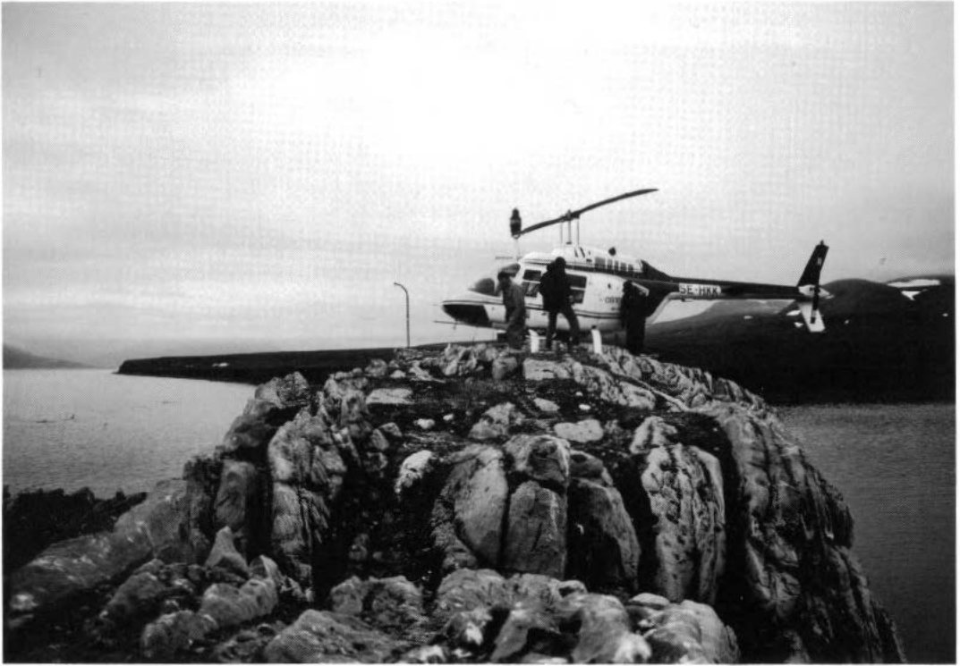
Helicopters may be used in the lighthouse maintenance work performed by the Norwegian Polar Research Institute. Photo: N. G. Flaata
