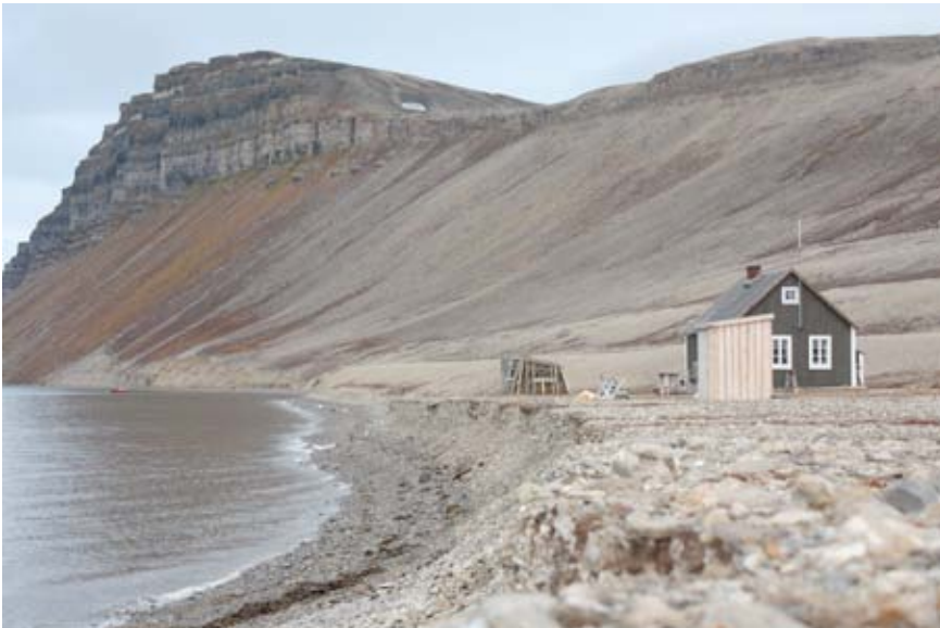
Fredheim by Sassenfjorden. Coastal erosion brought the sea 11 metres closer to the main building between the first measurement in 1990 and September 2009. Danielbu, in the background, is the oldest building at the station. In 2001, this hut was moved several metres northeast from its original site when the encroaching shoreline came too close. All photos by the author.
