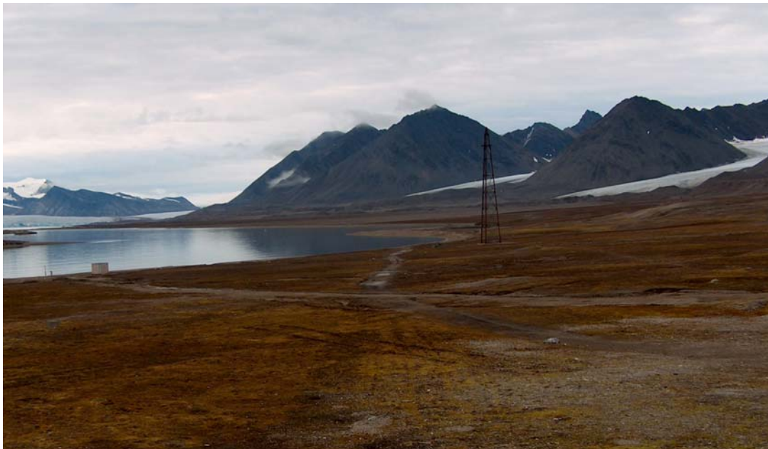
Figure 8.6. Path leading to the Amundsen mast. Photo: Gunnar Sander.
