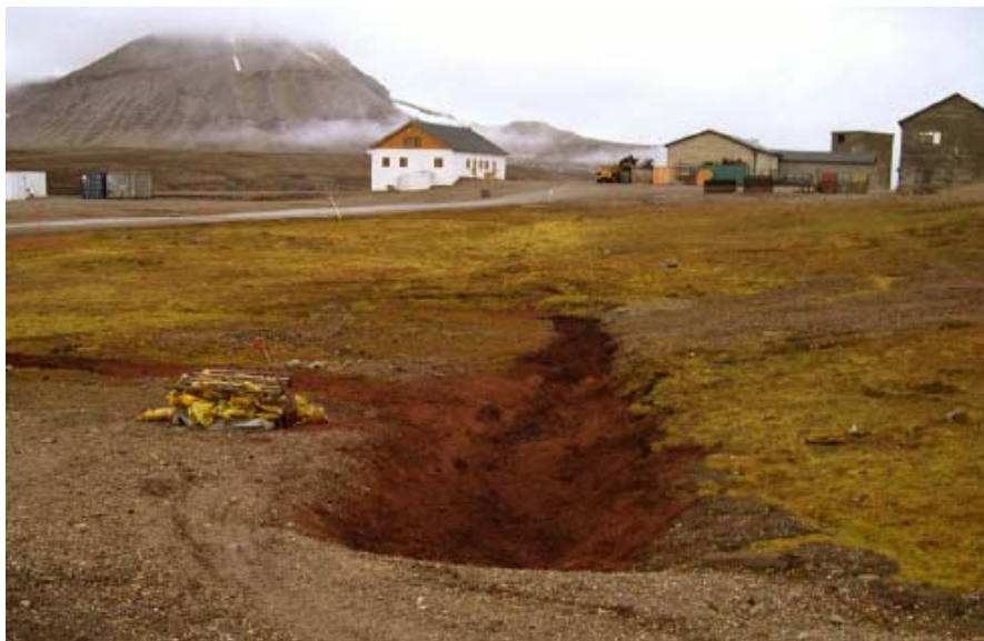
Figure 6.2: Closure of the ditch below the fuel tanks. The brown colour is from an oil absorbant. Photo: Kjell Tore Hansen.
