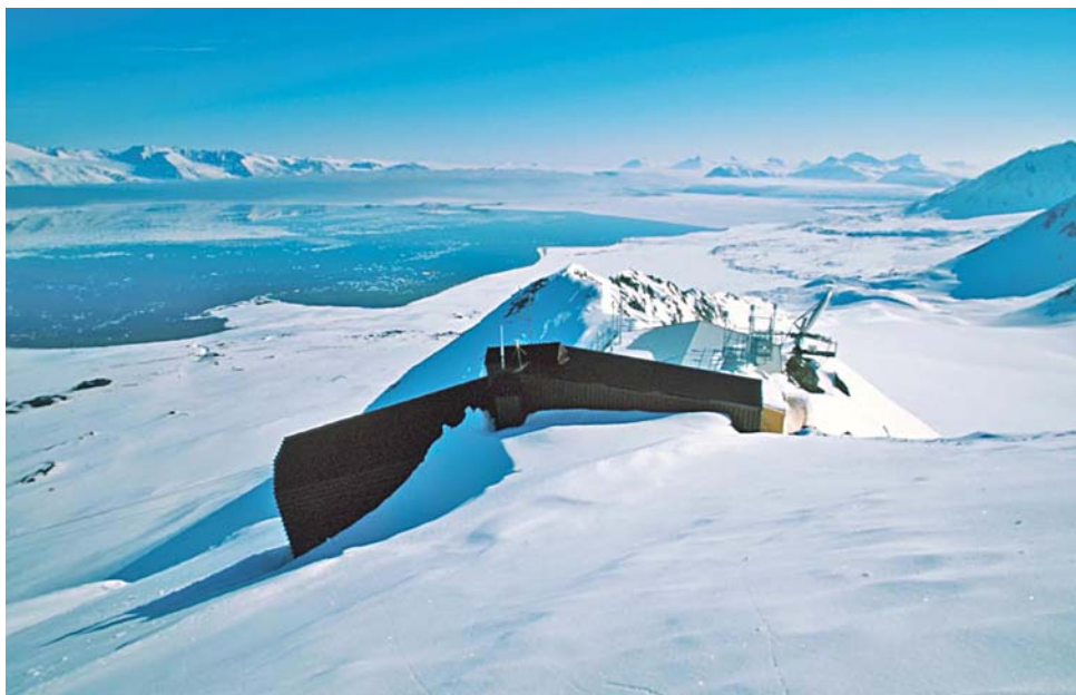
Figure 8.4. Zeppelin Station. Photo: Tor Ivan Karlsen.
