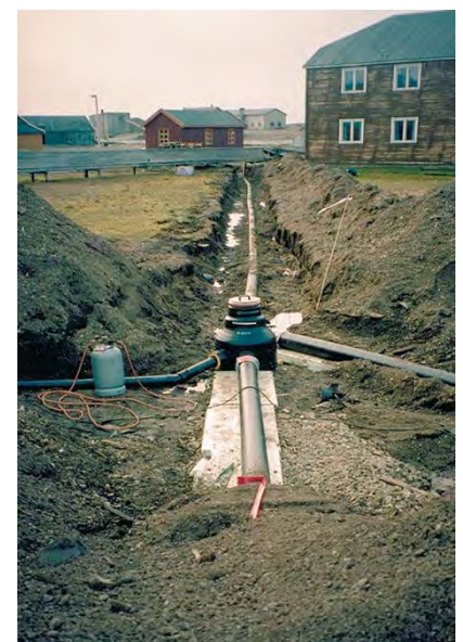
Damage to tundra due to underground burial of pipelines and services. Photo: J. Shears (BAS).
