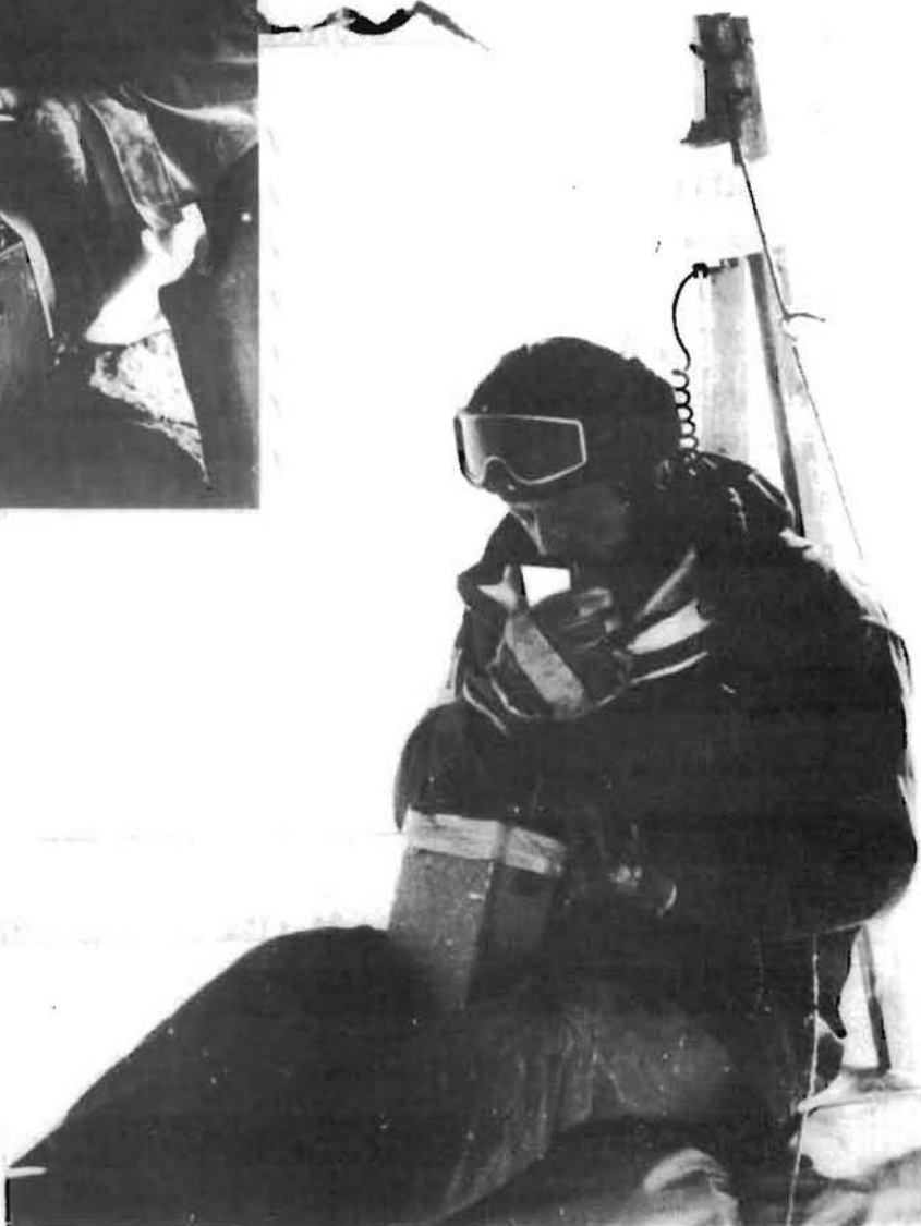
Fig. 2. Tape recording of magnetometer measurement. Note position of magnetometer sensor above the head of the operator.
