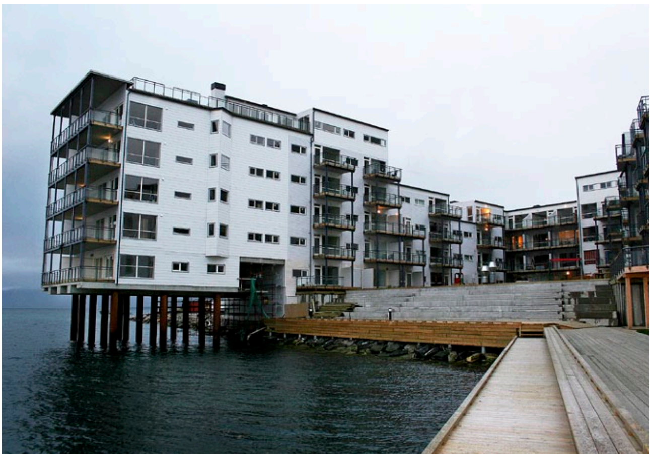
New housing complex constructed on landfill just above sea level. Tomasjordnes in Tromsø. Image: © Torgrim Rath Olsen, Nordlys
