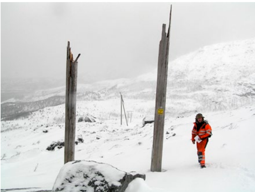
The electricity supply failure in Steigen municipality in January 2007, which affected 1097 households, 134 commercial customers and 587 cabin owners and left them without electricity for almost six days, is an example of how older and/or poorly maintained electricity supply infrastructure can be vulnerable to extreme weather. Strong winds were the cause of direct damage to power lines and pylons, these were also indirectly damaged by falling trees, causing a breakage of power network cables. Image: © Nord-Salten Kraftlag
