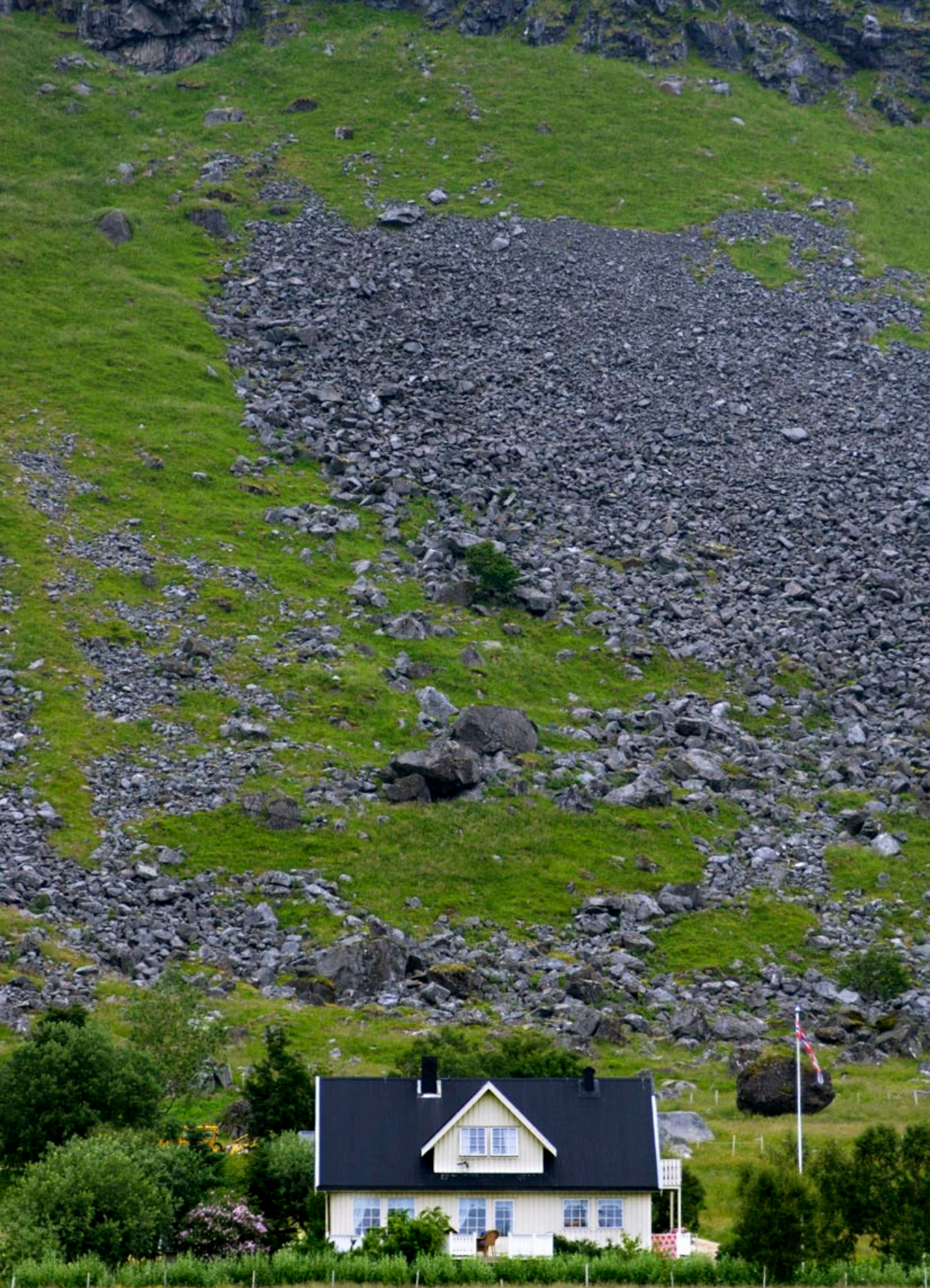
Villa in an area prone to landslides, Vestvågøy municipality, Lofoten. Image: © Dag Røttereng, Samfoto
