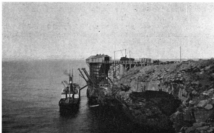
Fig. 55. Coal-pocket, Austervåg. Steamer (1 180 tons dw.) loading. Looking east. — G. Horn phot. 5/7 1924.
