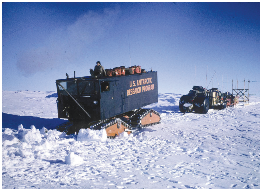
Figure 2 | Scenes from above the shores of the Recovery lakes. The 1965–66 US–UK South Pole–Queen Maud Land traverse, showing a Sno-Cat tractor and, in the background, a ‘rolly’ tyre set containing fuel, and the ice-sounding radar antennae. The tractor is just crossing a crevasse at the edge of the Recovery ice stream, near where Bell et al. 2 have now discovered four subglacial lakes.
