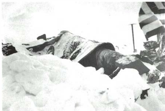
Fig. 43. Nansen's winter hut on Jackson Island, as found by Baldwin in 1902. The hut has been dug free of snow, and the walrus hides over the roof pole may clearly be seen. Photo: Anthony Fiala.
