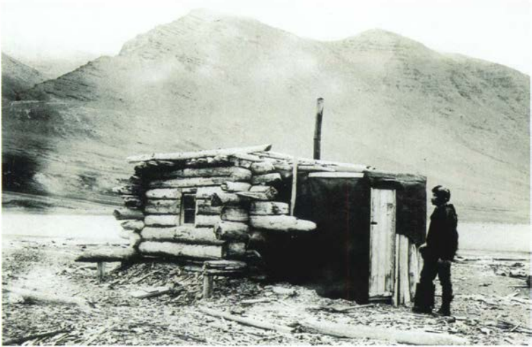
Fig. 87. A trapper's hut at Krosspynten (Wijdeffjorden) photographed by Adolf Hoel's expedition in August 1912. Two trappers had spent the previous winter there. One had died of scurvy and was found by the expedition members, the other had just managed to struggle to Longyearbyen. The main hut is built of logs derived from driftwood, and resembles the huts which Russian trappers had constructed earlier.
