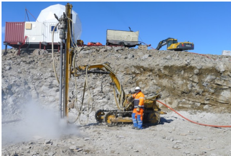
Boring for Tr. 3 antenna
