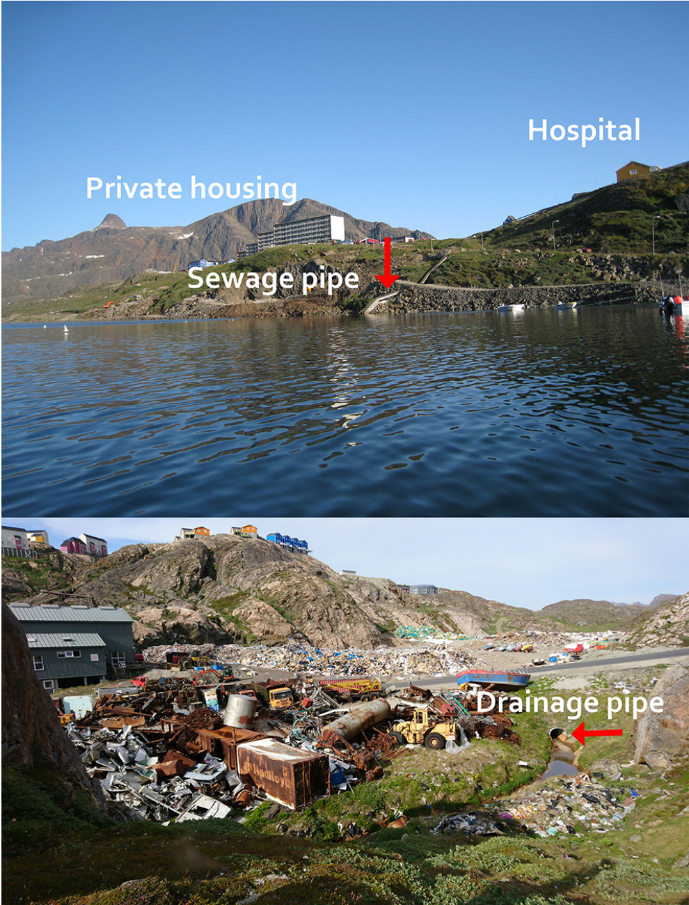
Figure 2: Wastewater outlet (sewage pipe) in Ulkebugt bay (top) and by the main dumping site with drainage pipe releasing waste leachate into the sea, Sisimiut (bottom).
