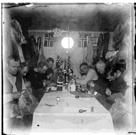
Inside Framheim at Whalers Bay in 1911. National Library of Norway.
