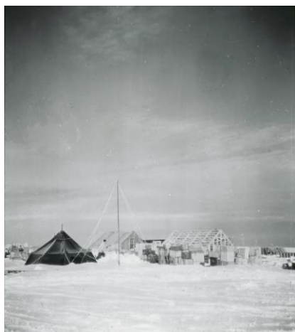
Maudheim under construction. Photo: V. Schytt, 1950. Norwegian Polar Institute's Photo Archives.
