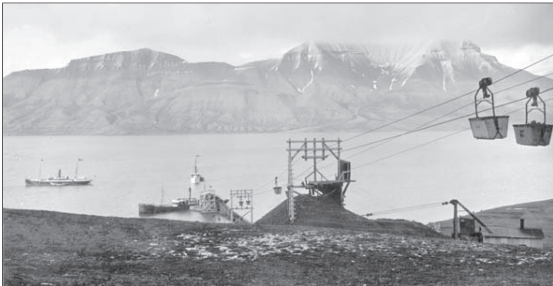
The cable-car was used for the transport of the coal from the mines to Longyearbyen and to the harbour.
