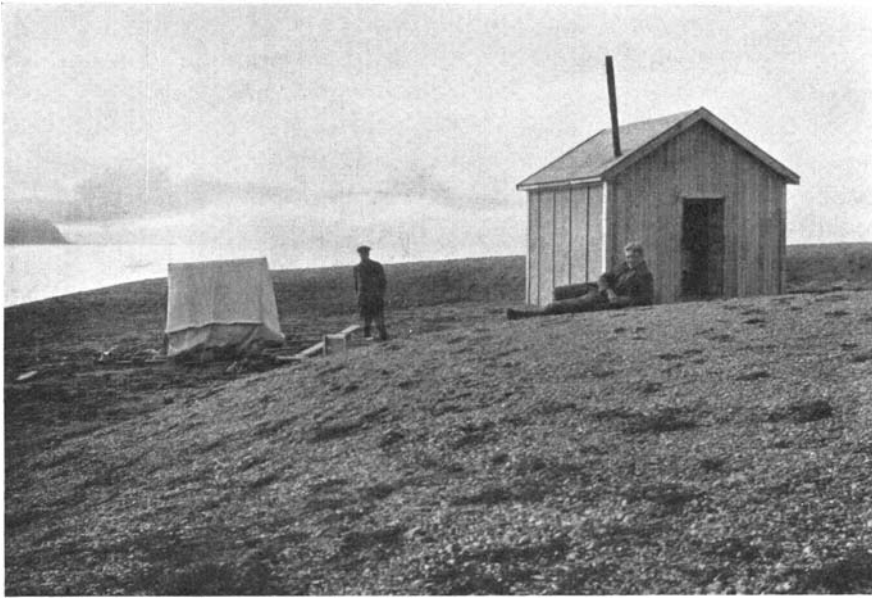
Fig. 49. Hut belonging to the mining company at Forlandsundet. L. J. Orvin phot. 9/8 1929.
